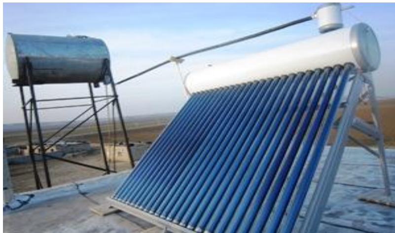
Figure 5-3 Installation of the first solar water heater system in Shahsevan winter camp site in Dasht-e-Moghan, Ardabil Source: http://www.ashayer-ar.ir
