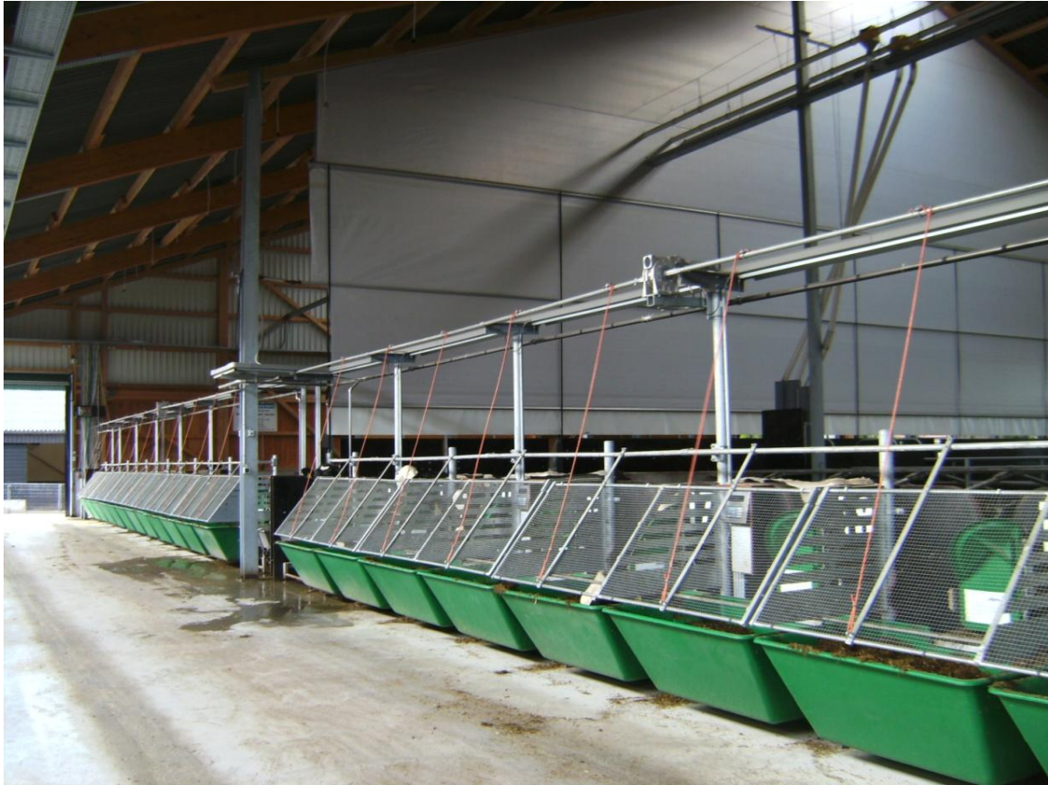
Figure 2.3 Foil partition of the investigated dairy barn
