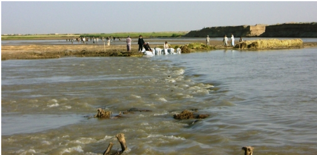
Photo P1: Flooded intake of Tarboz Guzar and Qal'a-ye Zāl irrigation canals
