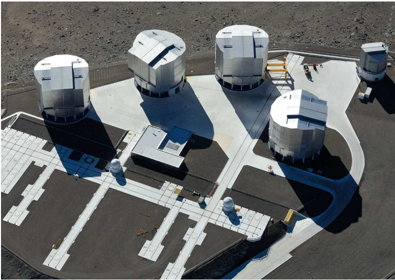
Figure 1.15: Photo of the Paranal platform with the four UTs and two of the ATs. The interferometric instruments are located in the VLTI laboratory in the building in the image center [Credit: ESO].
