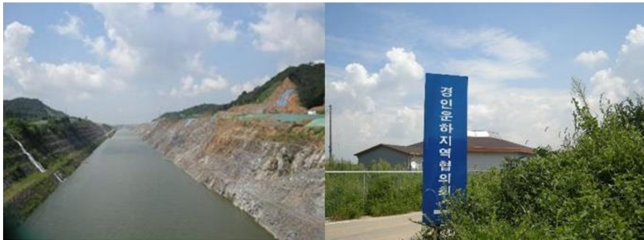
Figure 22 (22-1: Left) (22-2: Right): Gyeongin Canal construction site.
