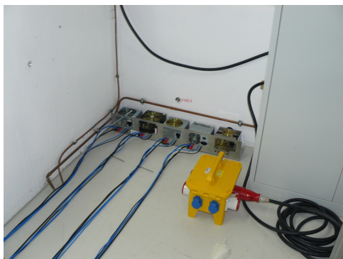
(e) Power supply units (standard ATX PC power supplies).
