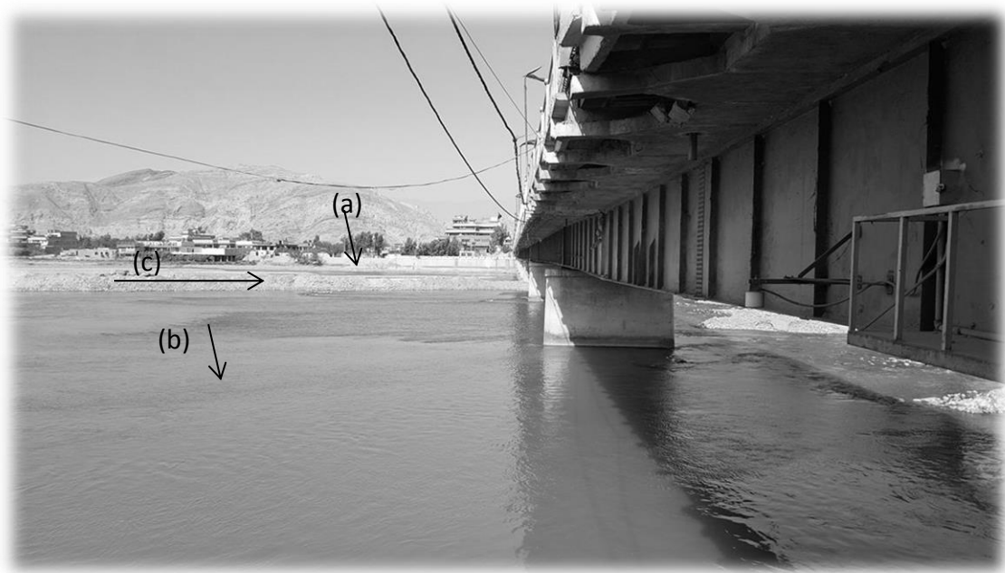
Figure 1.7: Streamflow divisions through temporary bifurcation and sand excavation along the river-bed while the staff gauge is installed at the far right along the cross section at Behsud Bridge on Kabul River; (a) and (b) are the two arms of the river as a result of the temporary bifurcation with the (c) sand piles in the middle of the river bed and causing the split of stream into two parts.
