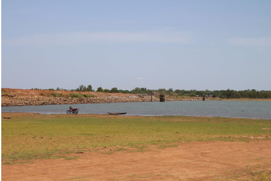
Picture 1. Vea Irrigation Dam
