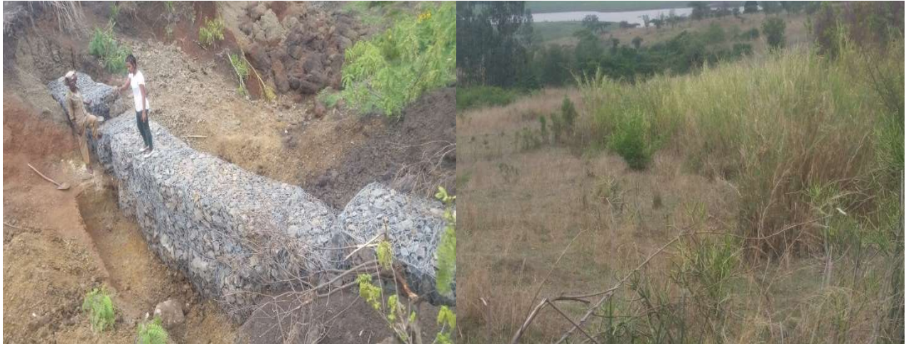
Figure 7. 3: Gully rehabilitation work (left) and rehabilitated gully (right) around the buffer zone
