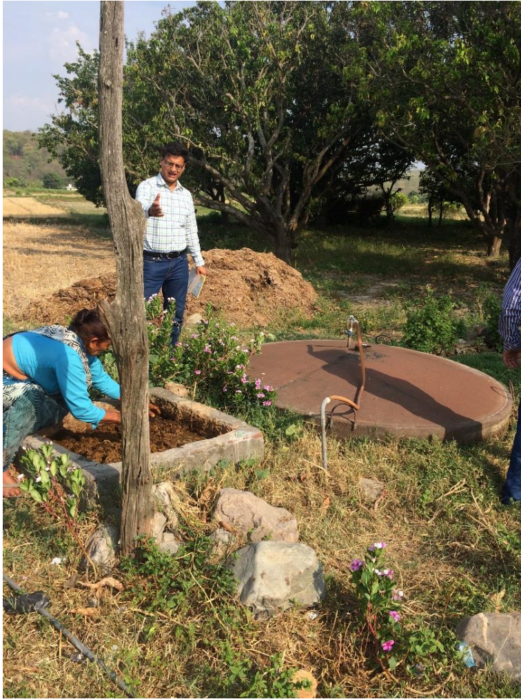
Figure 2.3: Field Observation- Operation of Biogas plant
