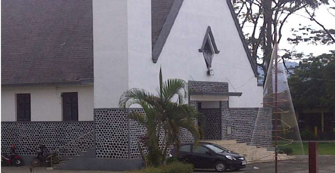
Figure 20: The oldest church in the Toraja regions located in Rantepao, North Toraja District Photo: Sukri, March, 2014
