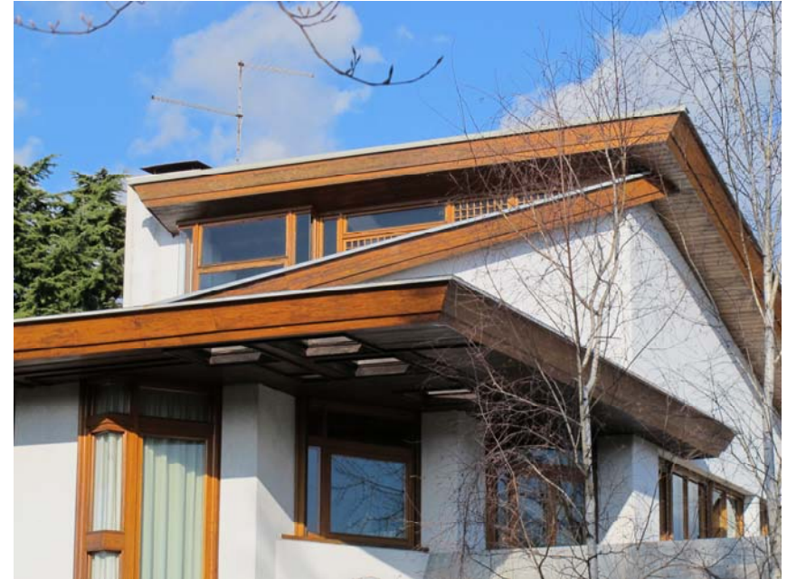
Abb. 91 Villa Romanelli, Detail des Attikageschosses
