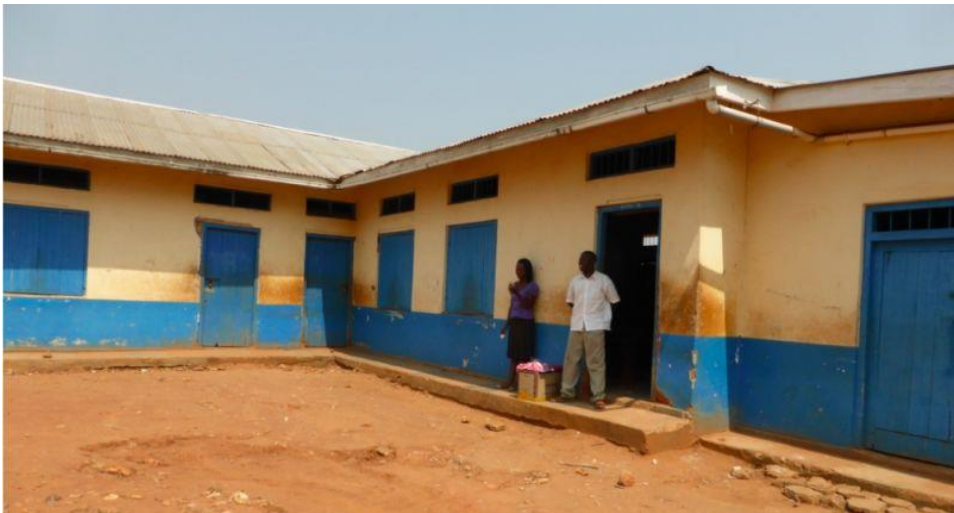
Photo 2.3-3: Sample site B - Primary school (Heinkel, 2015)
