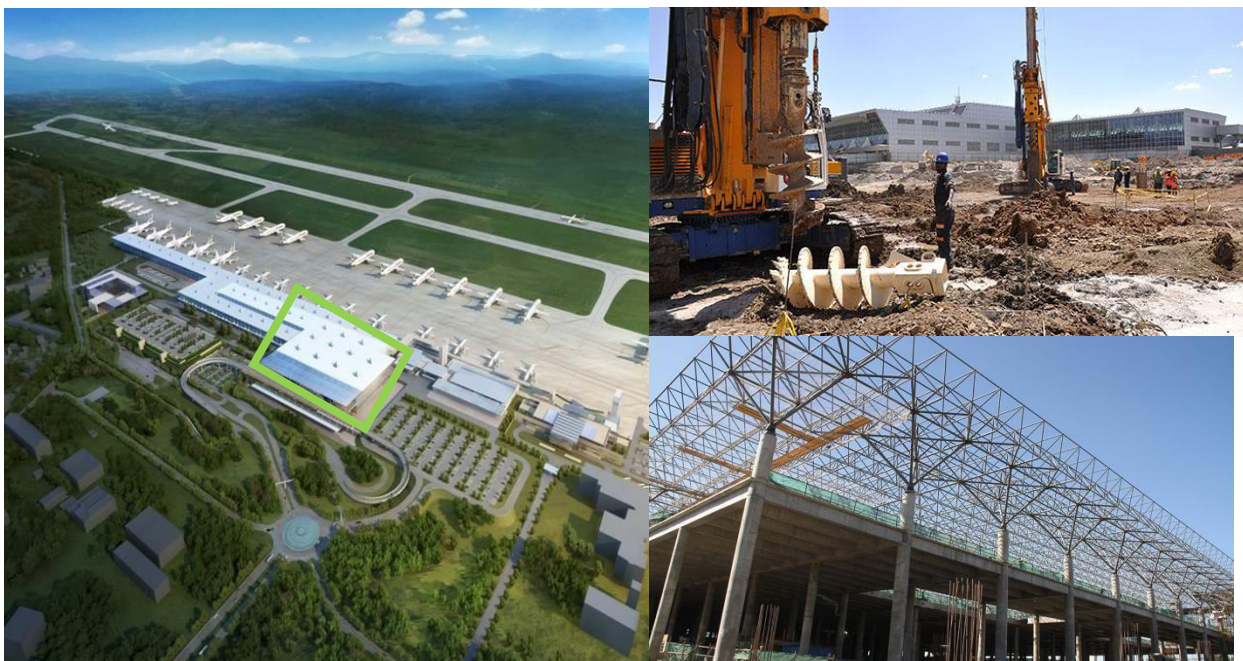
Abb. 171: Bole Expansion Project – Simulation (EAE 2014), Baustelle 2015/16 (ABDU 2015, KALEYESUS 2016s)
