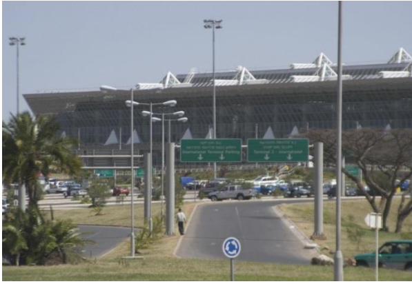
Abb. 52: Addis Ababa Bole International Airport Land-side (AABIA 2013)
