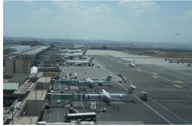
Abb. 53: Addis Ababa Bole International Airport Airside (EATCA 2017)
