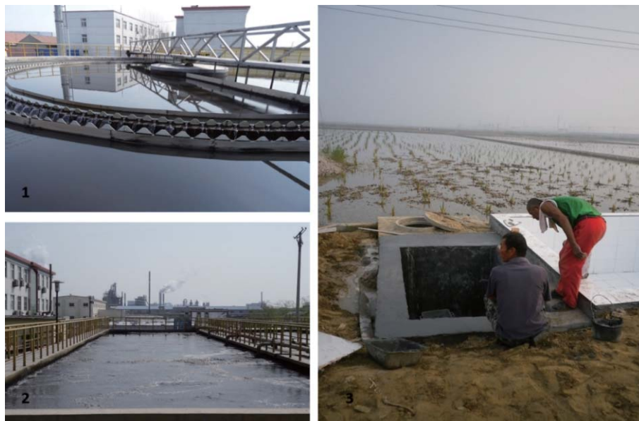
Photograph 2.2 Construction of WWT plants and constructed wetlands
