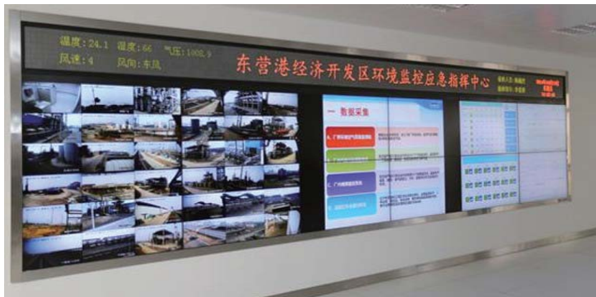
Photograph 2.1 The Environmental Monitoring Emergency Support Centre
