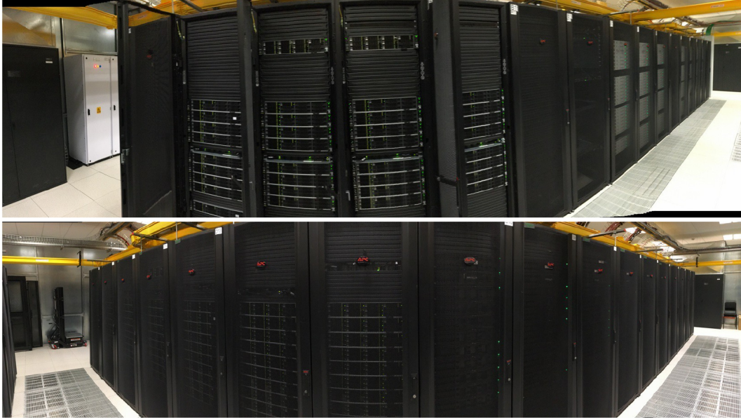
Figure 3.2: A fish-eye view of the TRAPUM user supplied equipment (USE) at the KAPB. Top panel is the FBFUSE rack. Bottom panel shows APSUSE consisting of 7 racks from the left with the rest belonging to TUSE. (Credits: E. Barr)
