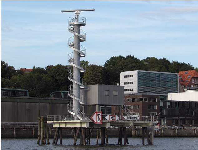
Figure 2.2: VTS radar tower in Hamburg (Germany) (picture taken from the web, www.lightphotos.net/photos/index.php ).
