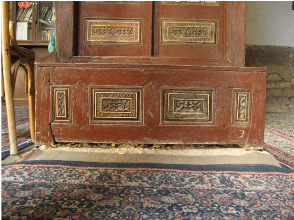
Minbar - Detail: Portal, Sockelzone
