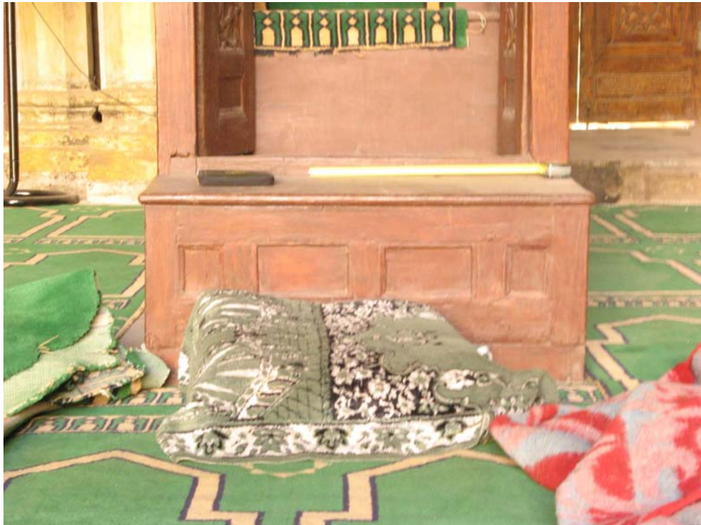
Minbar - Detail: Portal, Sockelzone
